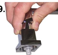
Complete the installation of your soap dispenser by screwing the trim on the brass fixing ring
